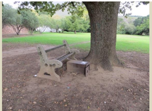
Figure 19 Unmaintained street furniture
