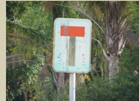
Figure 16 faded traffic sign
