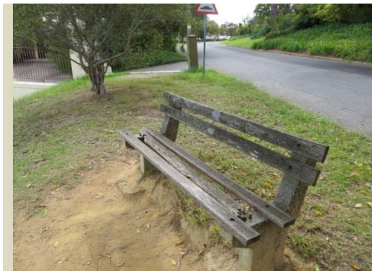
Figure 18 Unmaintained street furniture
