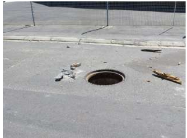
Figure 54 Some manhole covers are missing and created serious road safety issues
