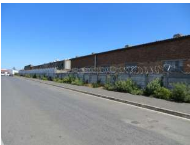
Figure 51 Some sidewalks are overgrown with weeds
