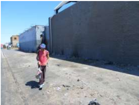
Figure 44 Poor sidewalk surface
