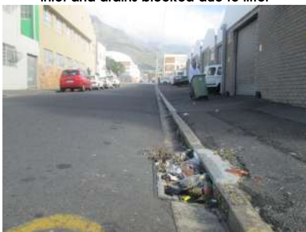
Figure 49 Storm water drains are blocked due to poor cleaning of streets
