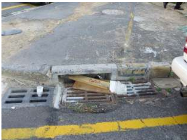
Figure 47 Some sidewalks and roads show curb inlet and drains blocked due to litter
