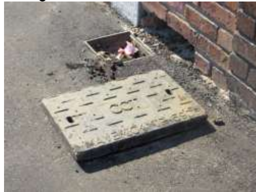
Figure 44 manhole on sidewalk without proper cover
