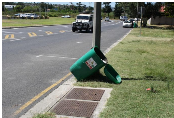
Figure 45 Broken infrastructure such as public phones shows neglect of certain aspects.
