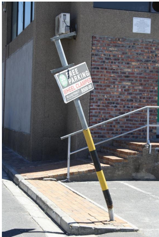
Figure 35 Bent and damaged sign
