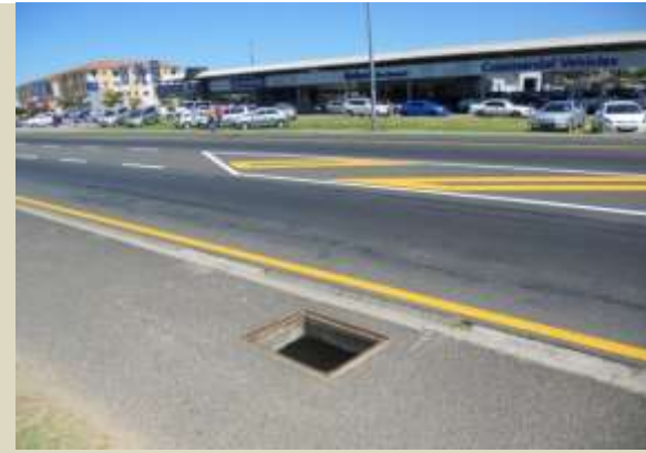
Figure 18 Broken manhole covers on sidewalks
